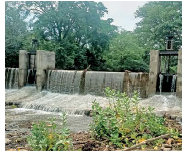
Water retention in check dams constructed on natural streams in MM Hills Wildlife Sanctuary, Karnataka.
